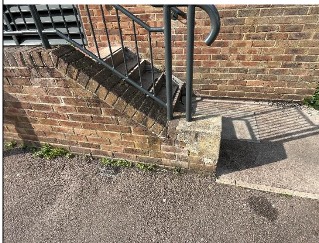
Figure 037: External rear elevation cracking to masonry
